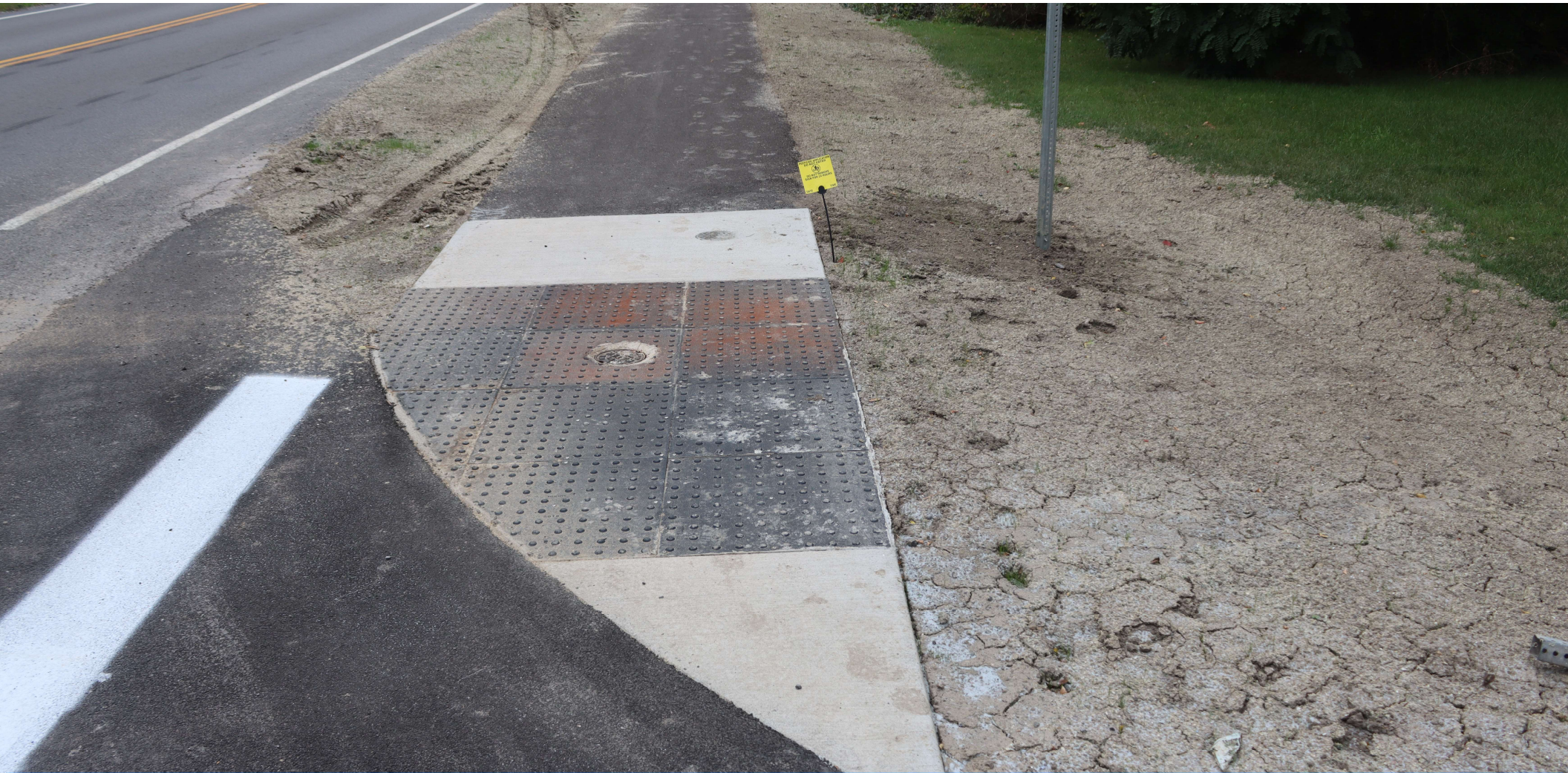
ADA RAMPS WITH CONCRETE CONTRAST AND TRUNCATED DOMES -- NOTE STRAIGHT ALIGNMENT, NARROW ALL CORNER RADII TO 25 FEET
