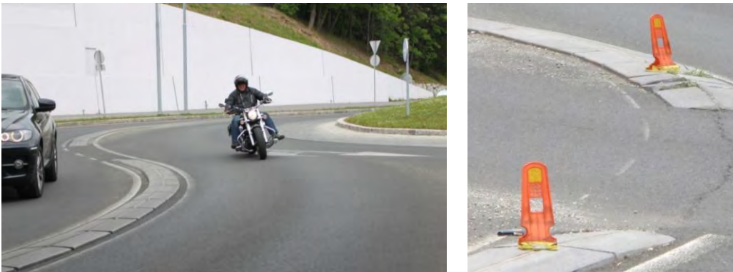
Figure 18. Flatter Raised Lane Divider in Slovenia and End Snow Markers (Tollazzi)
