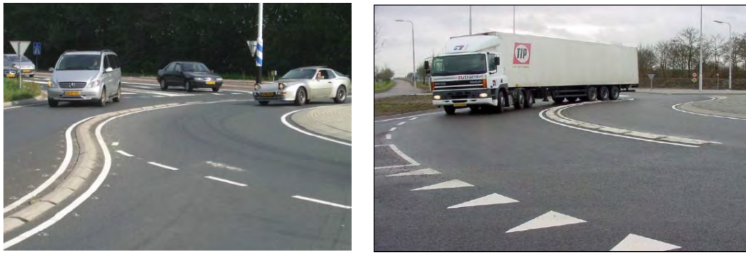
Figure 3. Turbo Roundabout Raised Lane Divider (Fortuijn)
